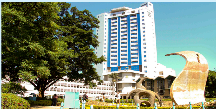
The University of Nairobi Towers at the Main Campus
